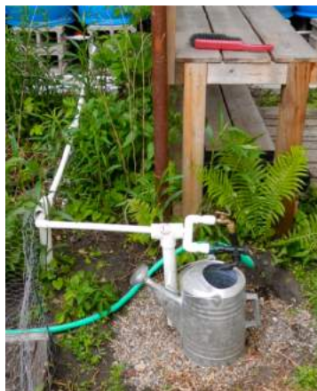
A home use, 350-gallon blue barrel interconnected rainwater collection system
